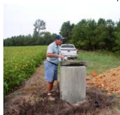
Well-capping South Centré Corridors
